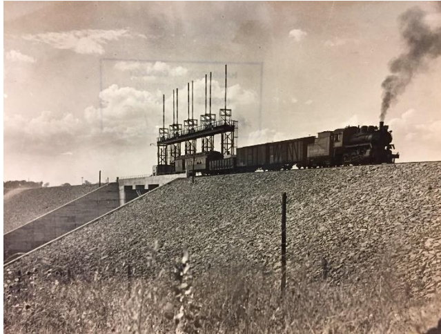
Fig 15.1 in Legget's and Paul Karrow's Handbook for Geology in Civil Engineering , published in 1983 by McGraw-Hill. The caption of this photo by Legget reads "The Shand Dam on the Grand River, Ontario, a dam built of glacial till with no core wall". Notice that Legget included a train in the photo.
