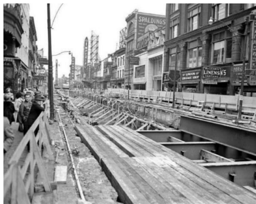
Toronto's Yonge Street subway under construction, using the cut and cover method of construction in the late 1940s (photo source City of Toronto Archives, Series 381, s0381_80015_id6207-3)
