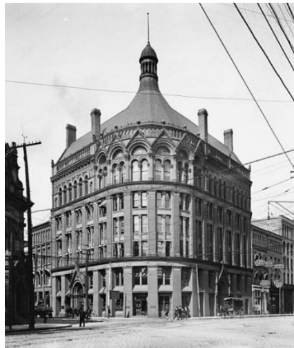
Early 1900s photo of the Toronto Board of Trade Building, head office of the TTC from 1921 to 1957 (photo source Wikipedia)
