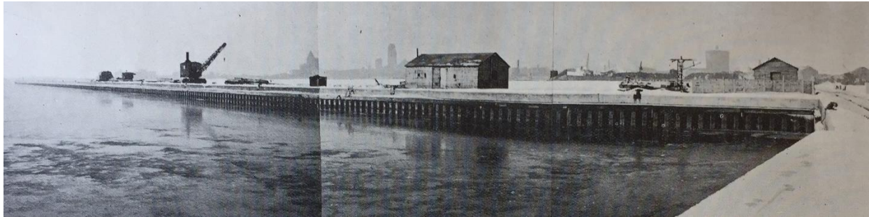
Panorama of the coal dock from Legget's article in Civil Engineering . Larsen sheet piling forms the facing of the dock. (LAC 4-60)
