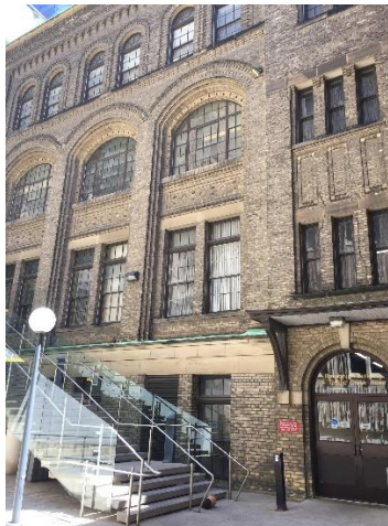
Basement entrance of the Electrical Building (Roseburgh Building). Legget's soil mechanics laboratory was in this basement. The staircase to the left leads to the Donnelly Centre opened in 2005. (photo Doug VanDine 2019)
